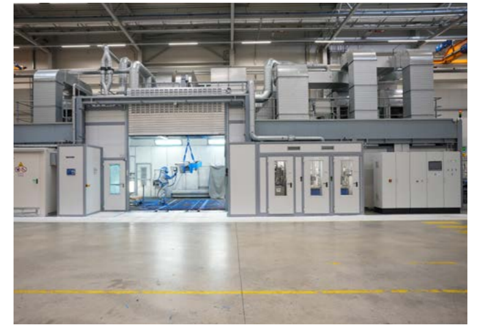
Corrosion protection and surface finishing using water-based paints
